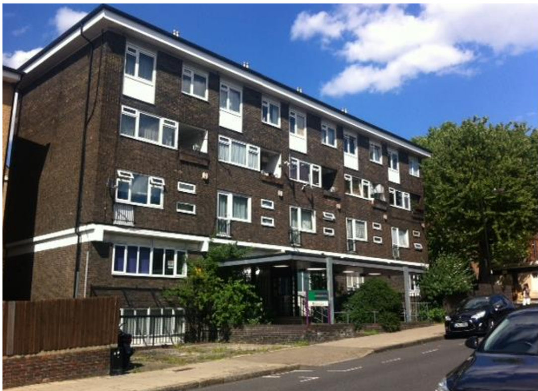
Photo 2: 1 Carnegie Street – subject site ground floor with residential units above
