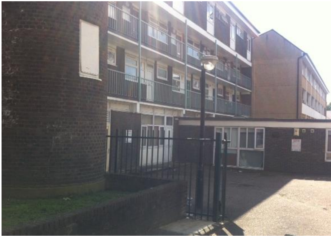
Photo 3: Rear of the building
